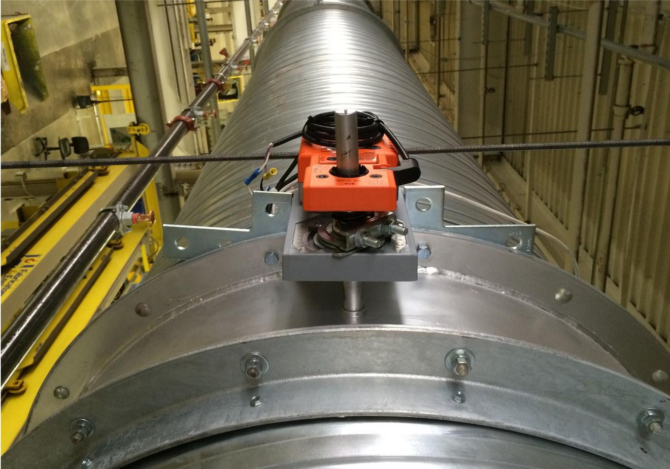
Belimo damper actuators are designed for use in a wide variety of HVAC applications for ensuring performance, reliability, and lower power consumption. Our comprehensive torque range (18 to 1,400 in-lb) is suited for damper sizes as small as 4-inch round allowing the ability to mount on standard damper shafts or directly on jackshafts. Actuators are used for control dampers, air handlers, economizer units, VAV terminal units, fan coil units, fan shutters, and unit ventilators.
